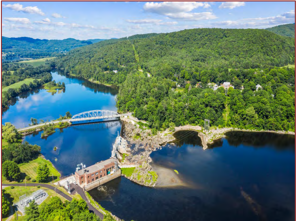
Figure 11: Downstream view of McIndoe Development 14
