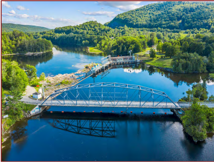
Figure 12: Upstream view of McIndoe Development 15
