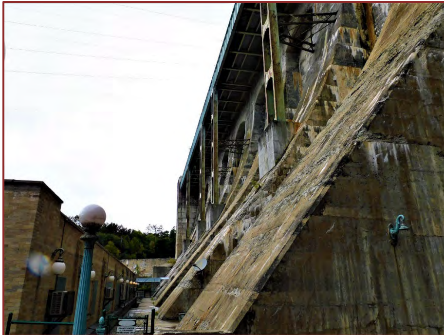
Figure 7: Comerford Station Dam
